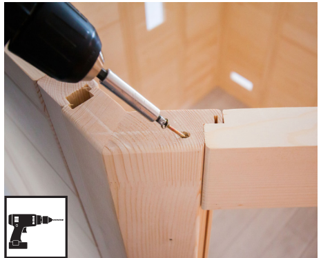
Foret de 3 mm, 1 vis 4 x 70 mm
