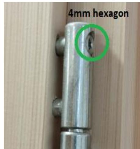
**Fig.2** Frame horizontal direction adjustment bolt
