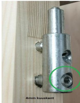
**Fig.3** Door sash depth adjustment bolt
