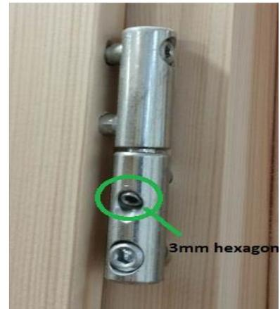
**Fig.1** Sash hinge height adjustment bolt
