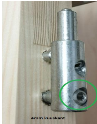
Fig.3 Door sash depth adjustment bolt
